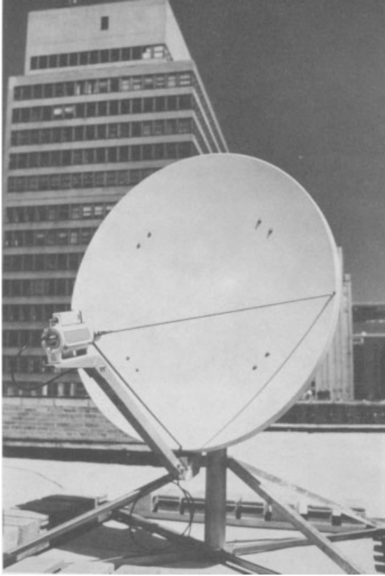
Figure 1.21 Photograph of the outdoor unit of a VSAT station. (Reproduced by permission of Gilat Satellite Networks, Ltd.)
